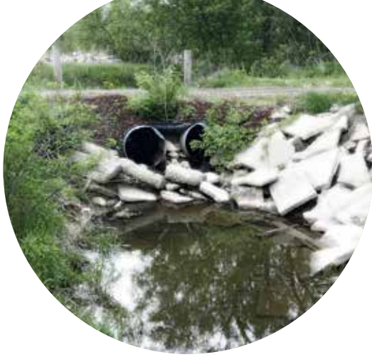
Somers Branch culvert replacement for fish passage and riparian improvements
