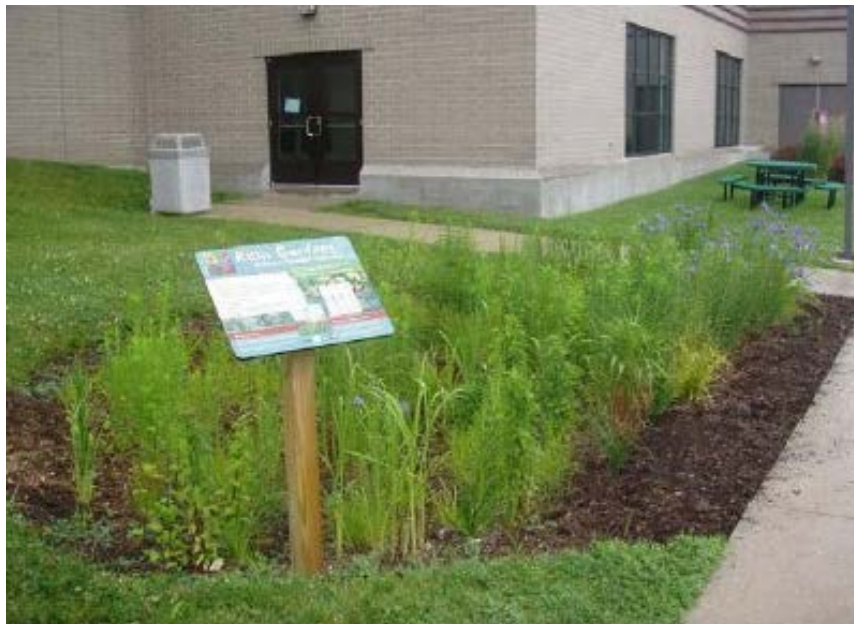
Improving green infrastructure - rain garden at Gateway Technical College in Racine. Source: Root-Pike WIN.
