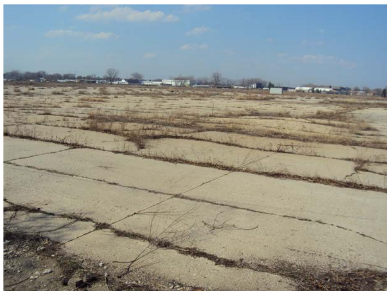
Remnant infrastructure at Case Brownfield Site (25A)
