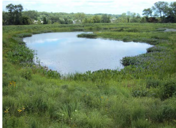
Properly designed wet bottom naturalized detention
