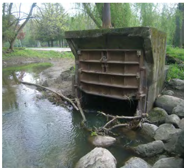
Dam at Petrifying Springs prior to removal in 2012.
