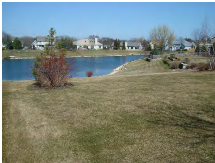
Typical wet bottom detention basin located southwest of Kr County Line Rd and County Trunk Highway Y.
