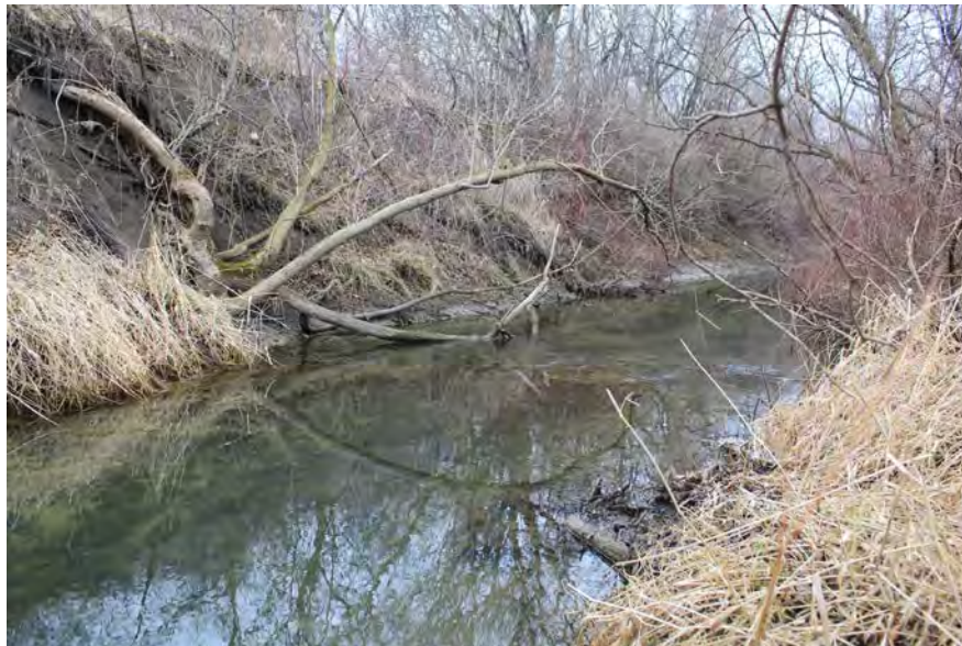
Excessive erosion along part of South Branch Reach 4
